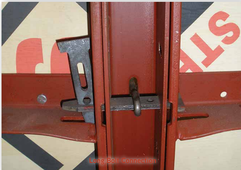
Typical Wedge Bolt Connection
